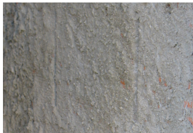
Preping the substrate with rough cast
